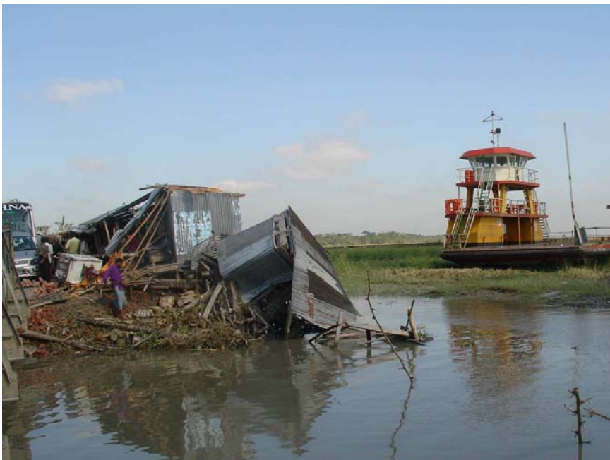
Facilities near a bridge and ferry crossing, badly damaged. Background shows a ferry washed ashore and grounded.
