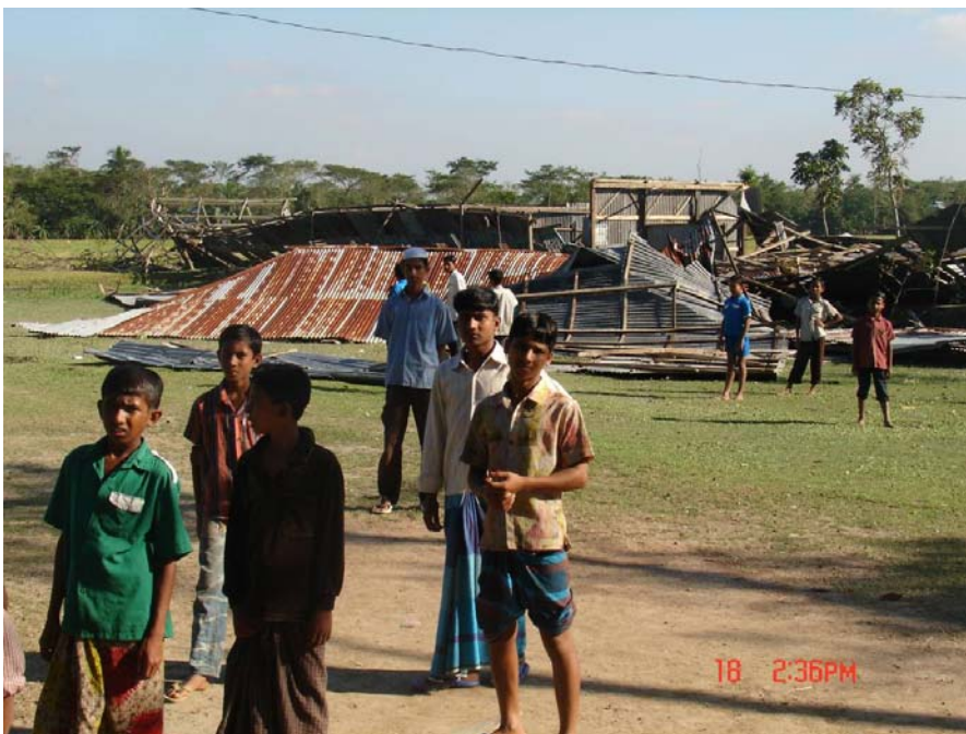
School children foreground, a flattened school building in the backdrop.
