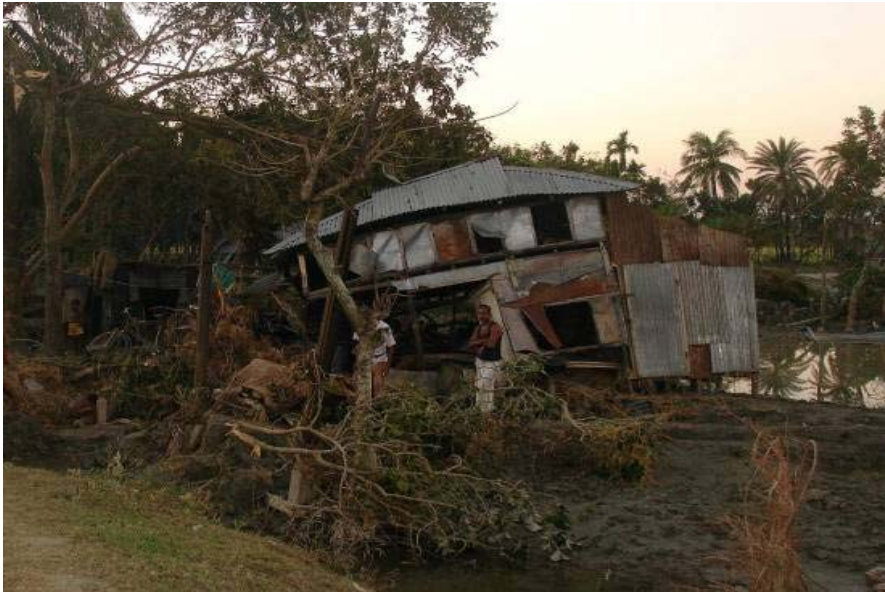
Badly damaged and leaning house located in close proximity to water.
